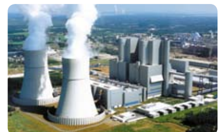
Fig. 2: Lignite power station "Schwarze Pumpe"
