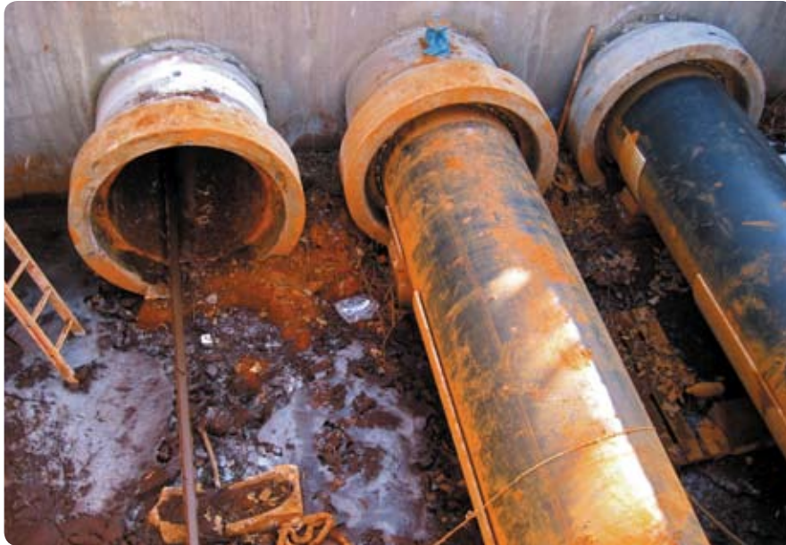
Fig. 7: Pipe lengths in an inspection shaft
