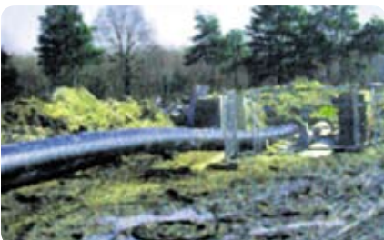
Fig. 4: Pipe length with pulling-in pit
