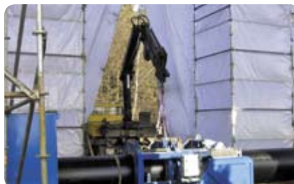
Fig. 6: Heating element butt welding machine with protective cover
